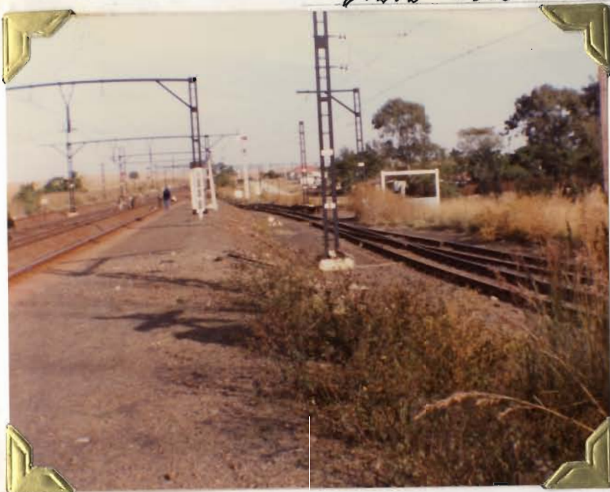
LEFT: The new Railway Line.
