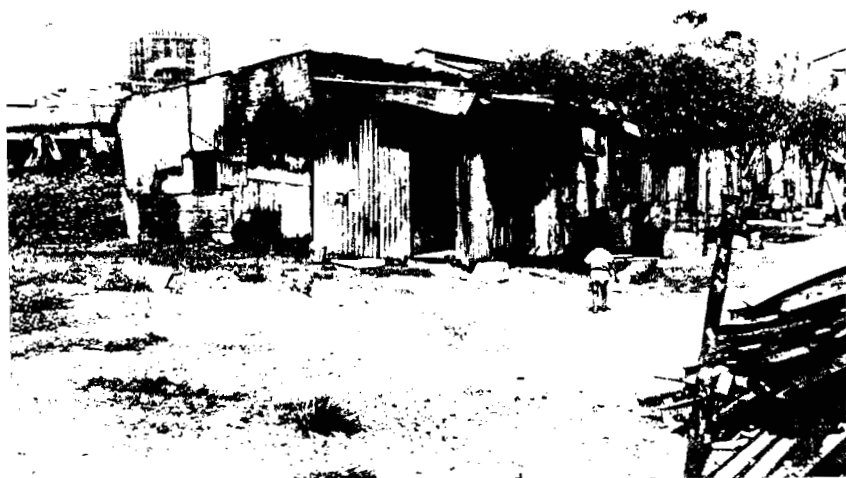
A TIN SHACK - SIMILAR TO THIS - BUILT BY LABOURERS.
