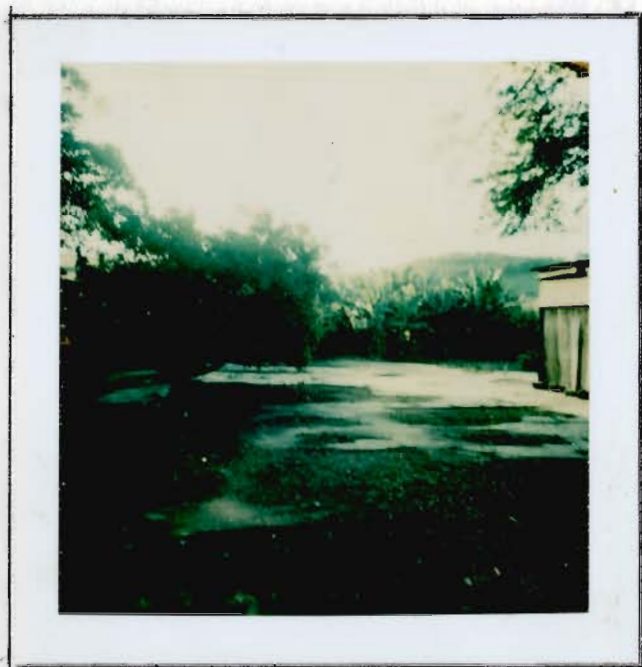
THE REMAINS FOUNDATION OF WHERE THE TEA FACTORY ONCE STOOD
