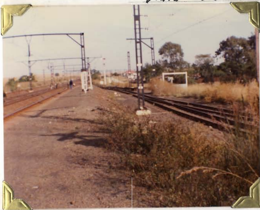
LEFT: The new Railway Line.
