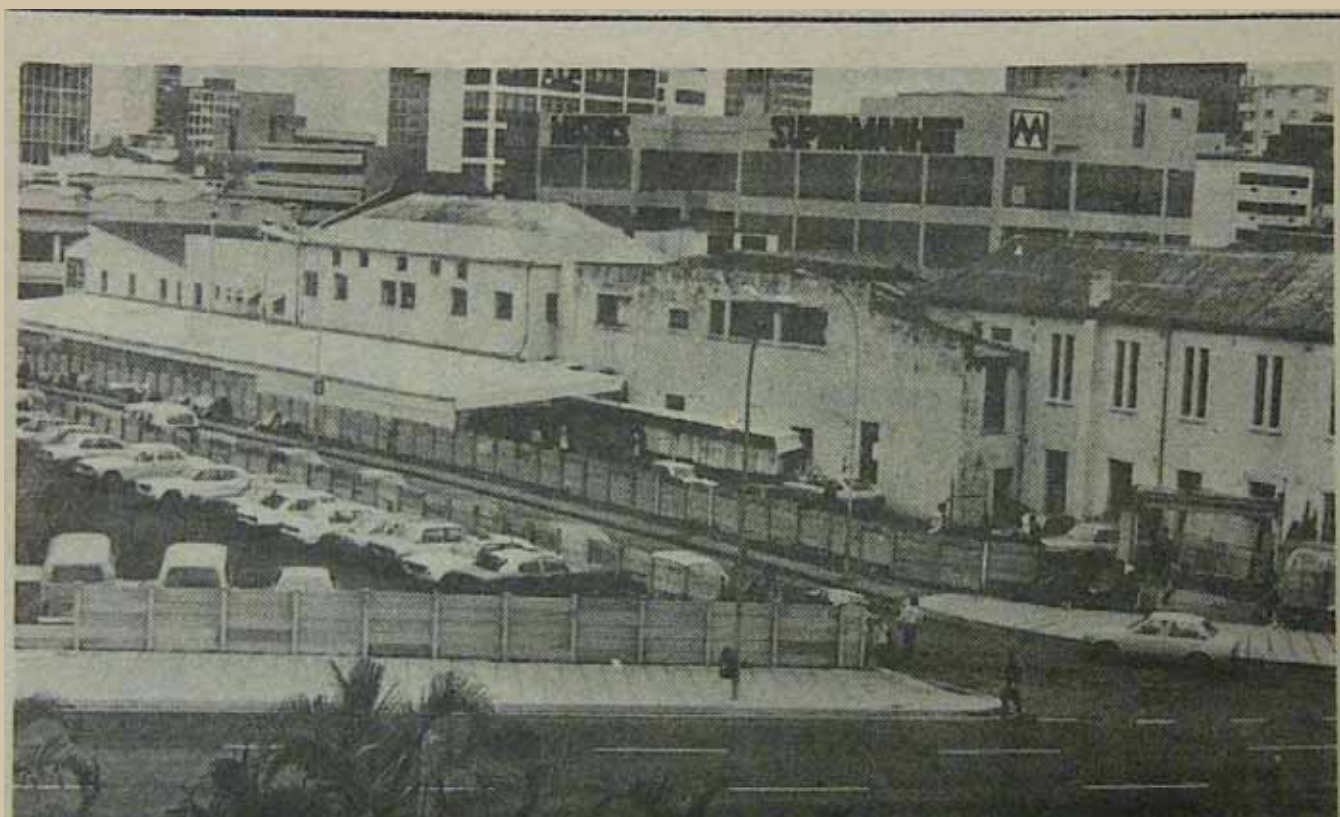
The vacant lot, once occupied by the market and the men's home, on the right, which is being offered to private developers.
