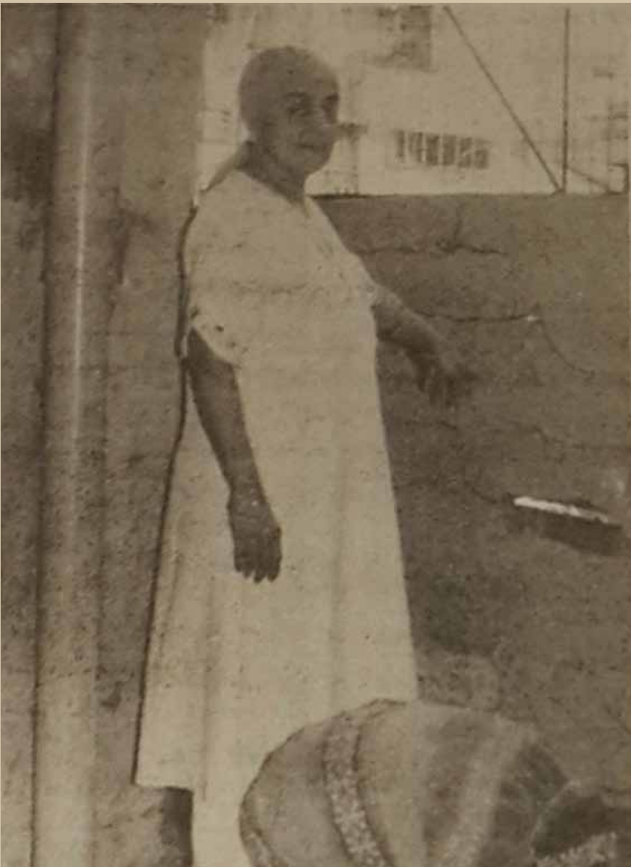
Juleika Moola, with some of her possessions, points to serious cracks in the wall, before leaving.
