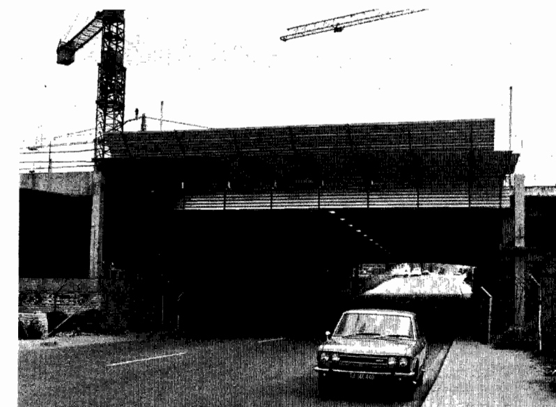
Avenue Road has been lowered to enable the Plaza to be built over it.
