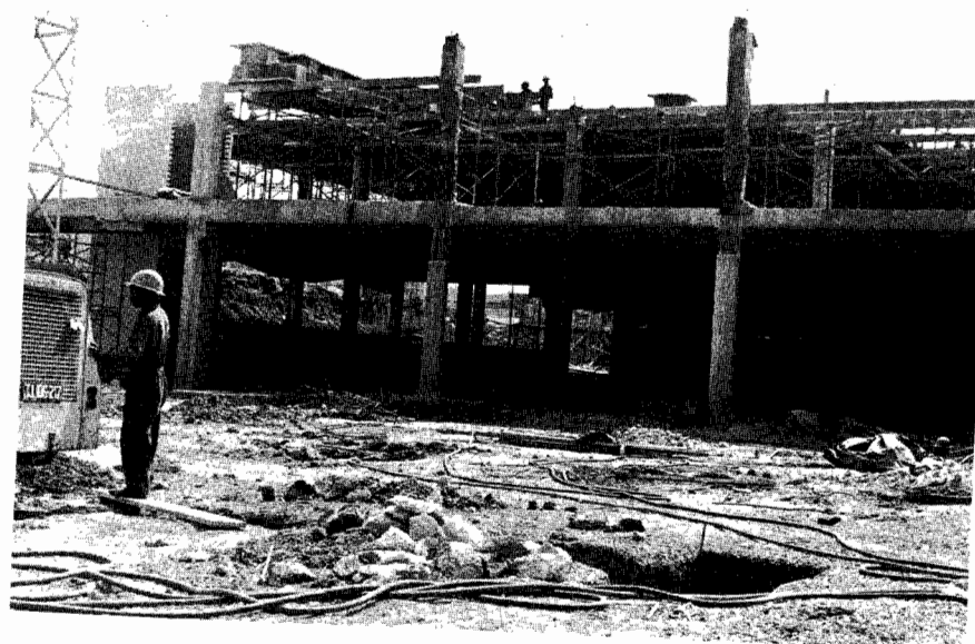
Construction work on the Western wing of the Plaza.
