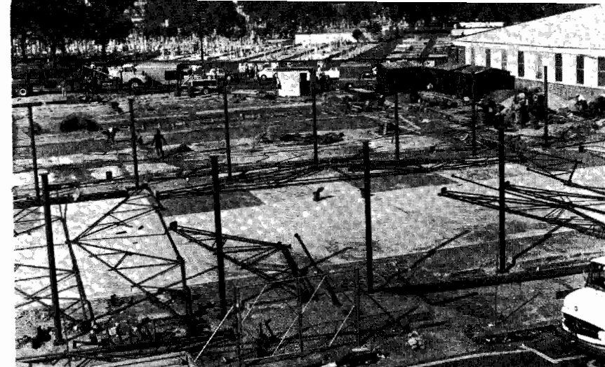
The site of the burnt out market cleared for reconstruction.
