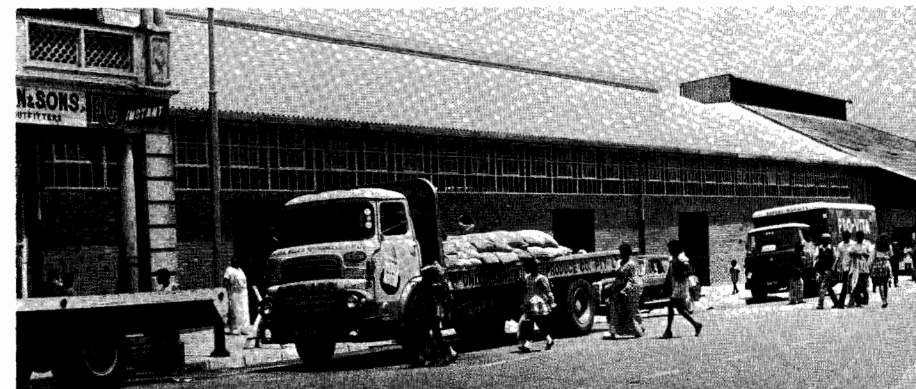
The newly-constructed temporary market buildings.
