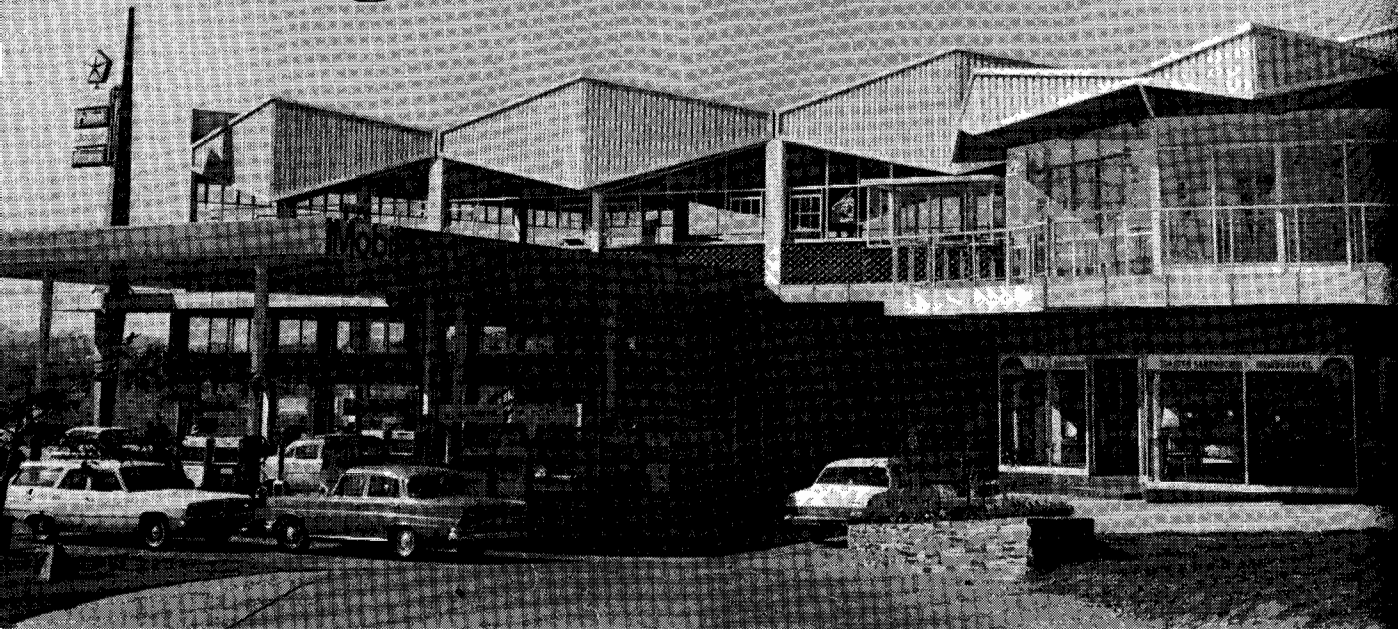
A view of the service station, the first floor workshop, and the café.
