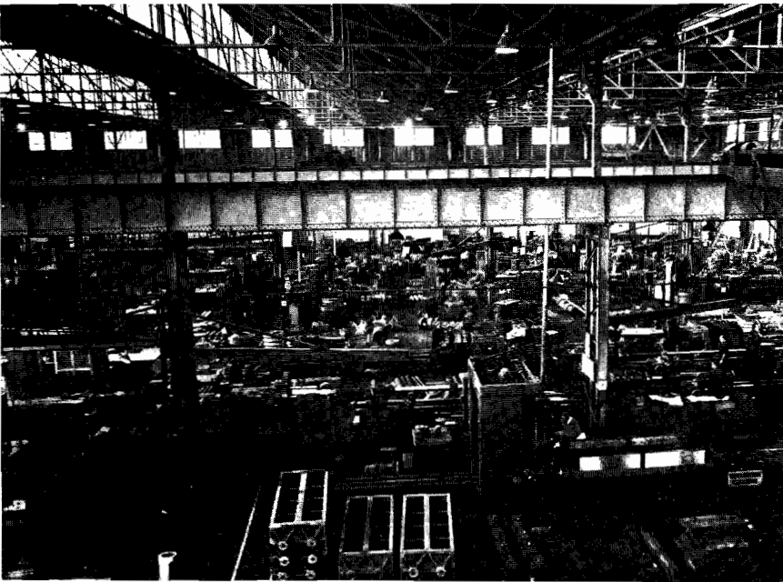
The partially completed Machine Shop building with the Main Stores building in the foreground.
