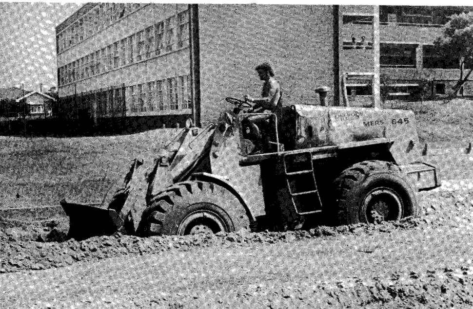
A tractor levelling the site for the new extensions to the College.
