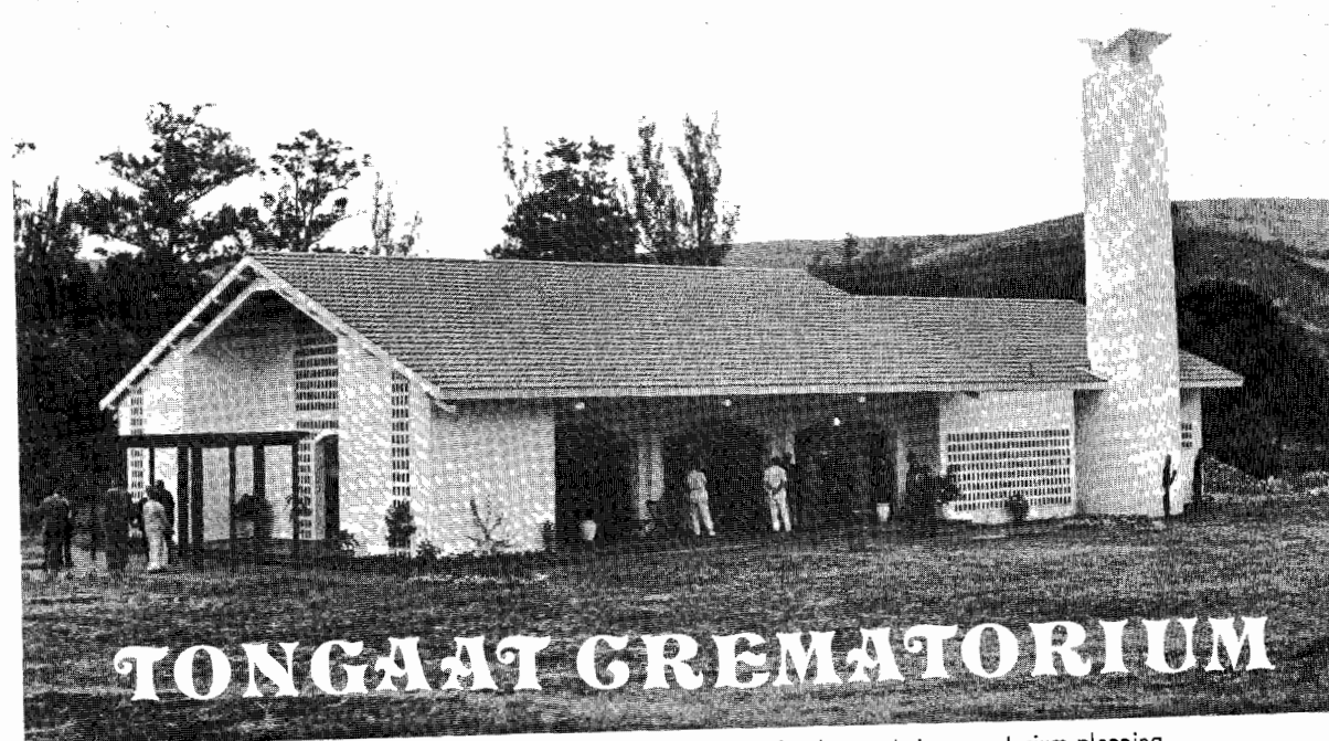
The new crematorium building incorporates the latest developments in crematorium planning.
