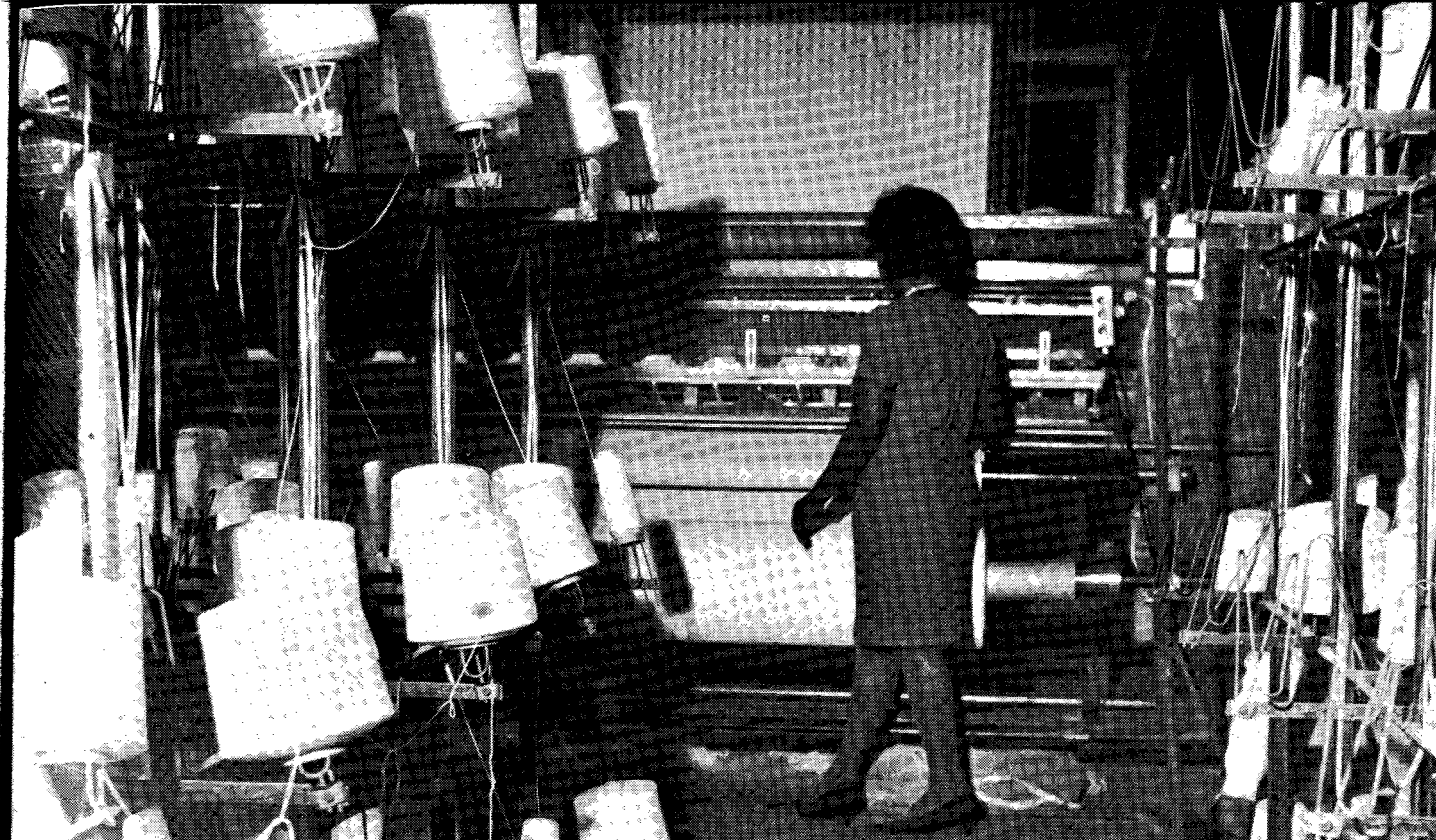
Bedspreads in the making. Thread from hundreds of spools is used on a base cloth of calico to produce the tufted effect of the well-known "candlewick" products.
