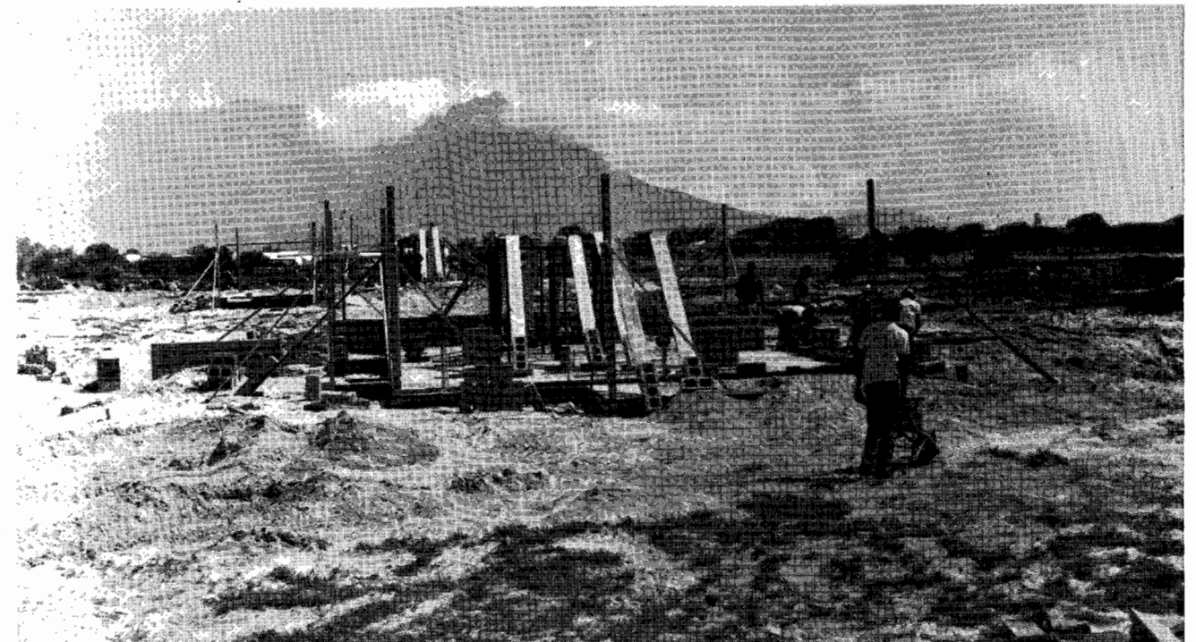
A panoramic view of the Cape Flats where 133 economic homes are under construction for Indian occupation. Table Mountain looms as a sentinel in the background.
