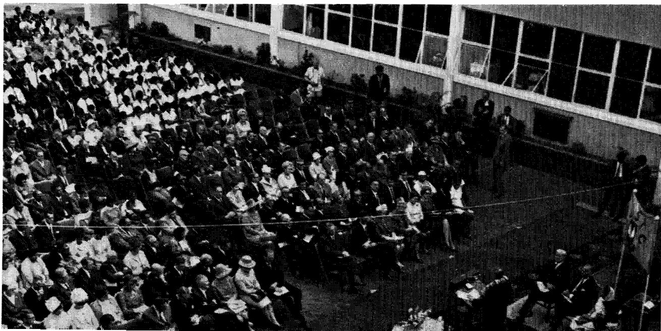
Below: Some of the large crowd and a section of the new block photographed during the Minister's address. A few minutes later Mr Waring unveiled the plaque at the lower right-hand side of the building and opened the door.
