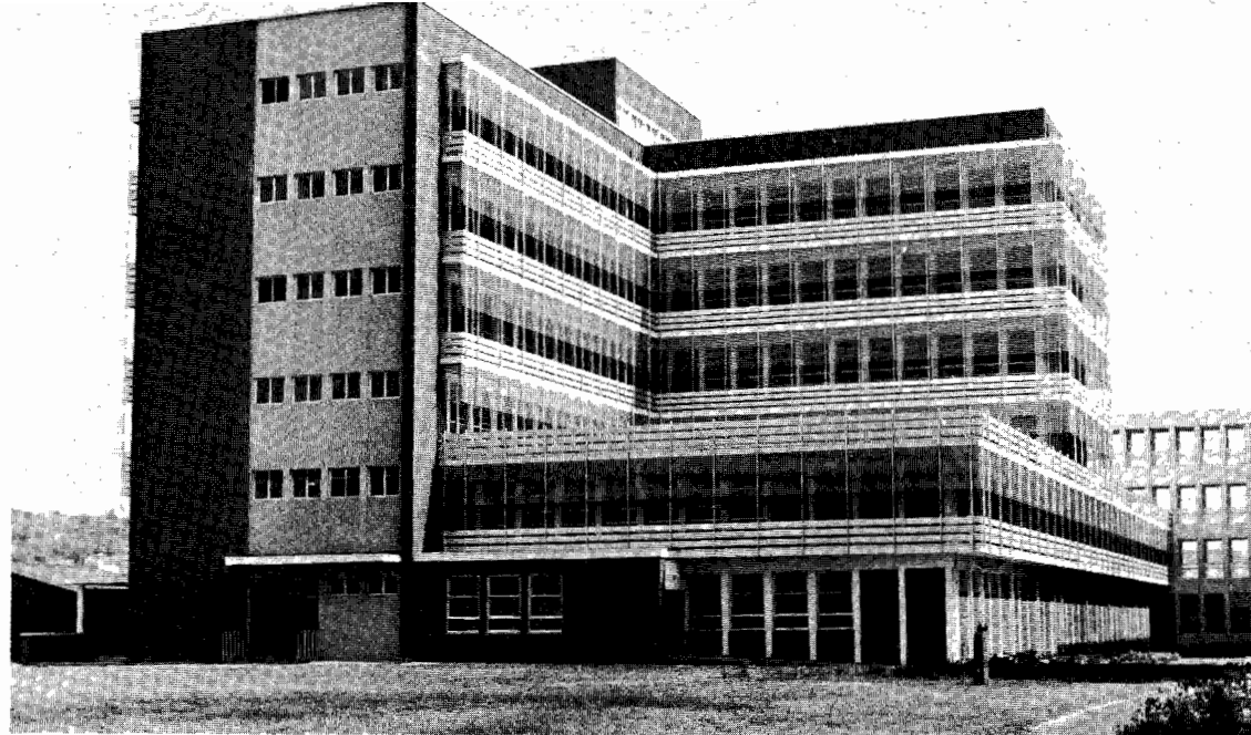
The new maternity block.
