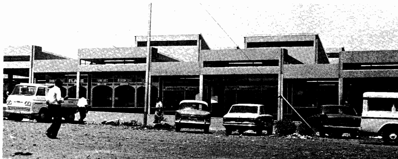
A view of the completed portion of the new shopping complex.
