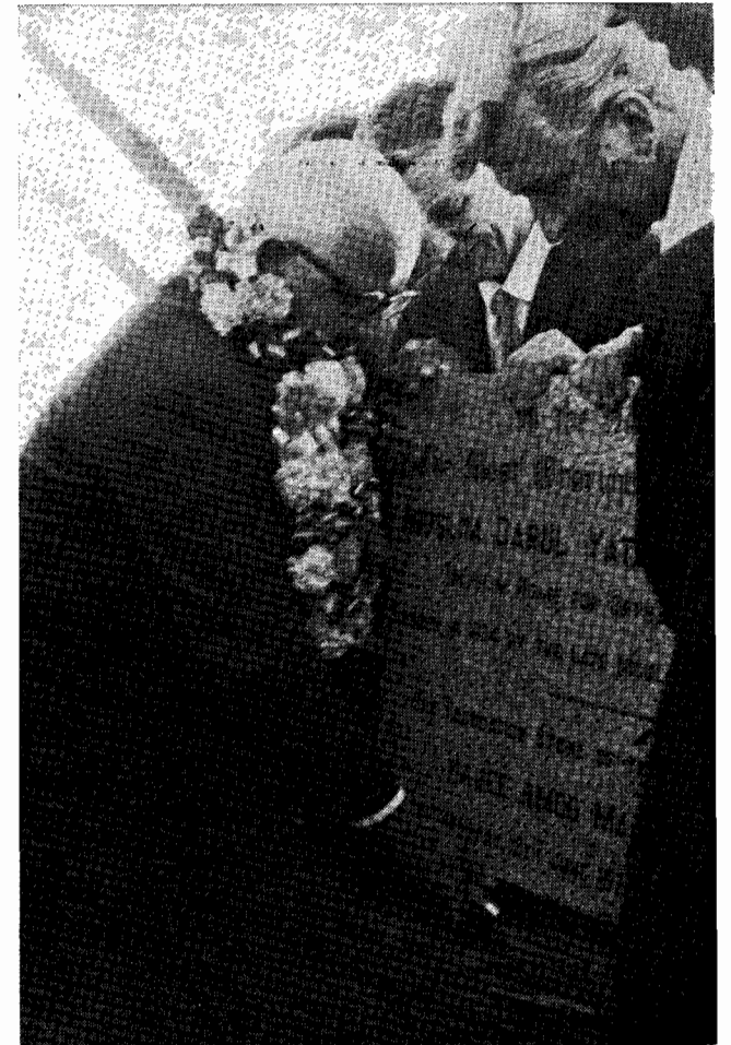
Mr A. M. Moolla is being assisted in the laying of the foundation stone by Mr Greening, the architect (right).
